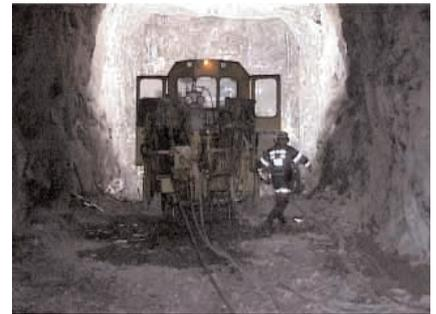
**Underground drilling rig extending the Lewis Decline, which was developed to facilitate exploration and provide access to new areas of mineralisation.**
