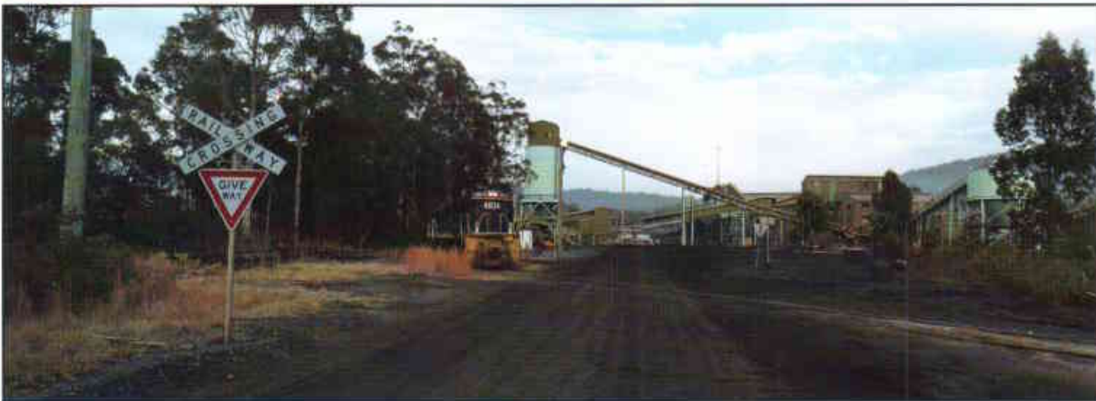
◀ The Southland Coal washing, storage and dispatch facilities.
